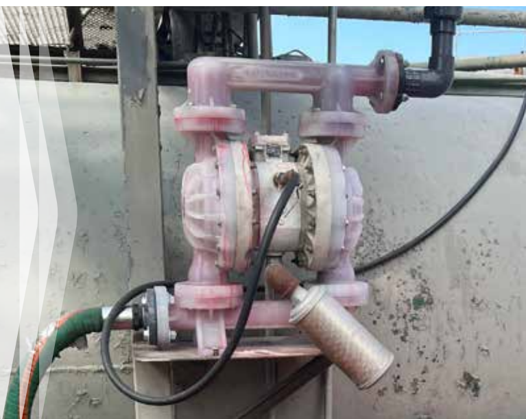
High suction lift reduces pump delivery.
