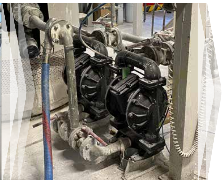
High fluid viscosity reduces pump delivery.
